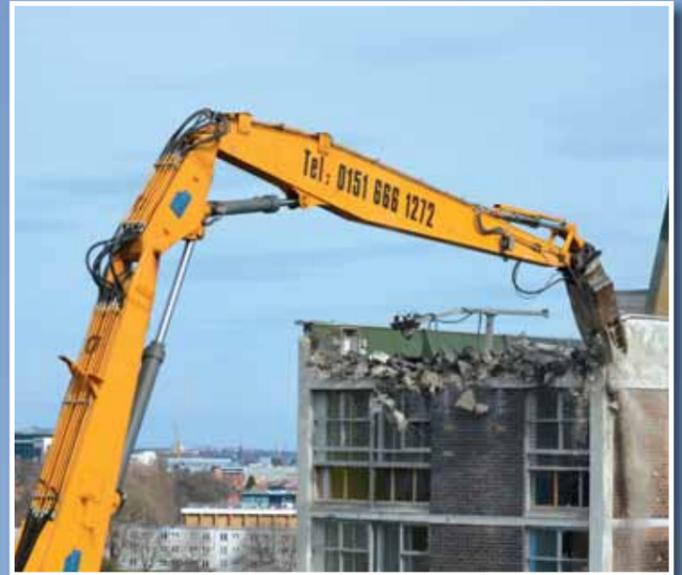
*Fully stretched to a pin height of 67m, the R984 can carry a 1.5t attachment. At 62m it can take a 2t tool, and much larger units with the three-stage boom retracted.*
